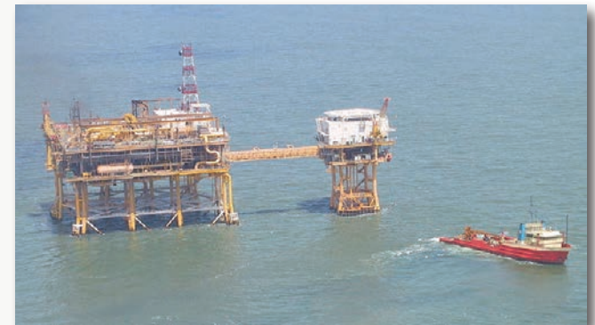
The Louisiana Offshore Oil Port (LOOP) is the only offshore deepwater port in the U.S. LOOP is connected to over 50 percent of the U.S. refinery capacity and has offloaded over 7 billion barrels of foreign crude oil since its installation ( http://loopllc.com ). Credit: Bob Webster
