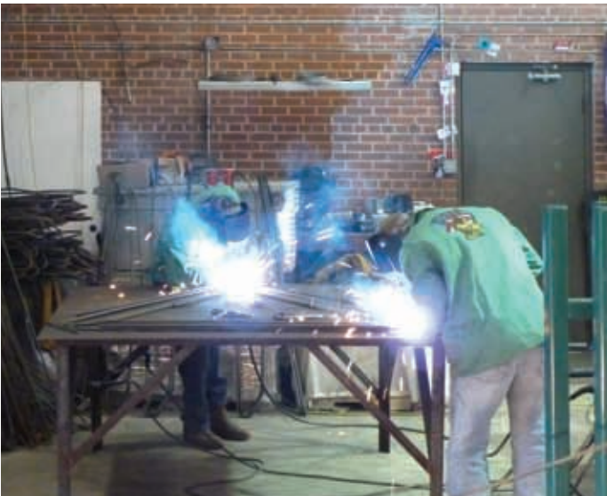
Welding to create the Reefblk© units. ©Richard Greig
