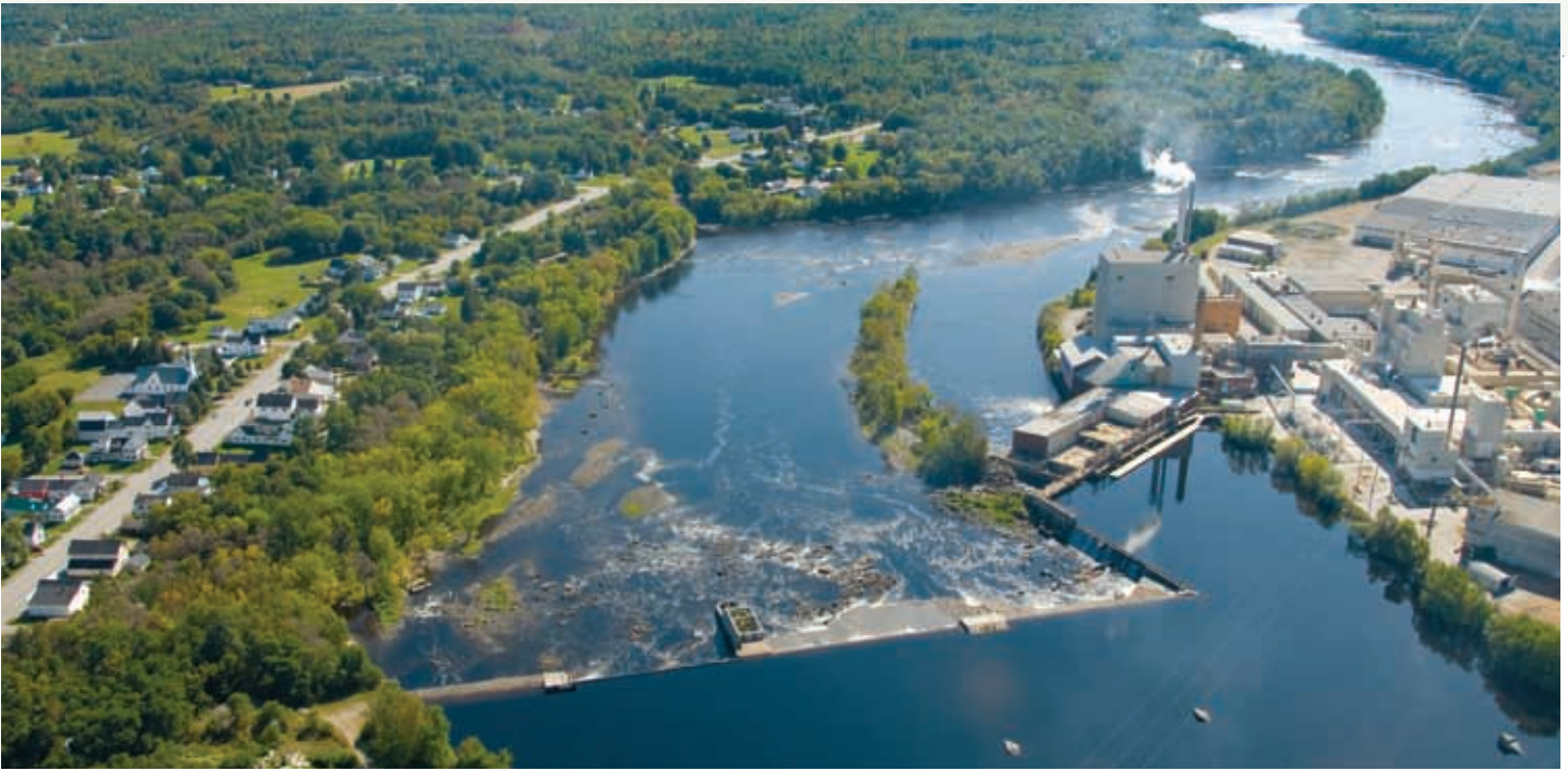
The Great Works Dam on the Penobscot River in the towns of Old Town and Bradley, Maine. ©Bridget Besaw
