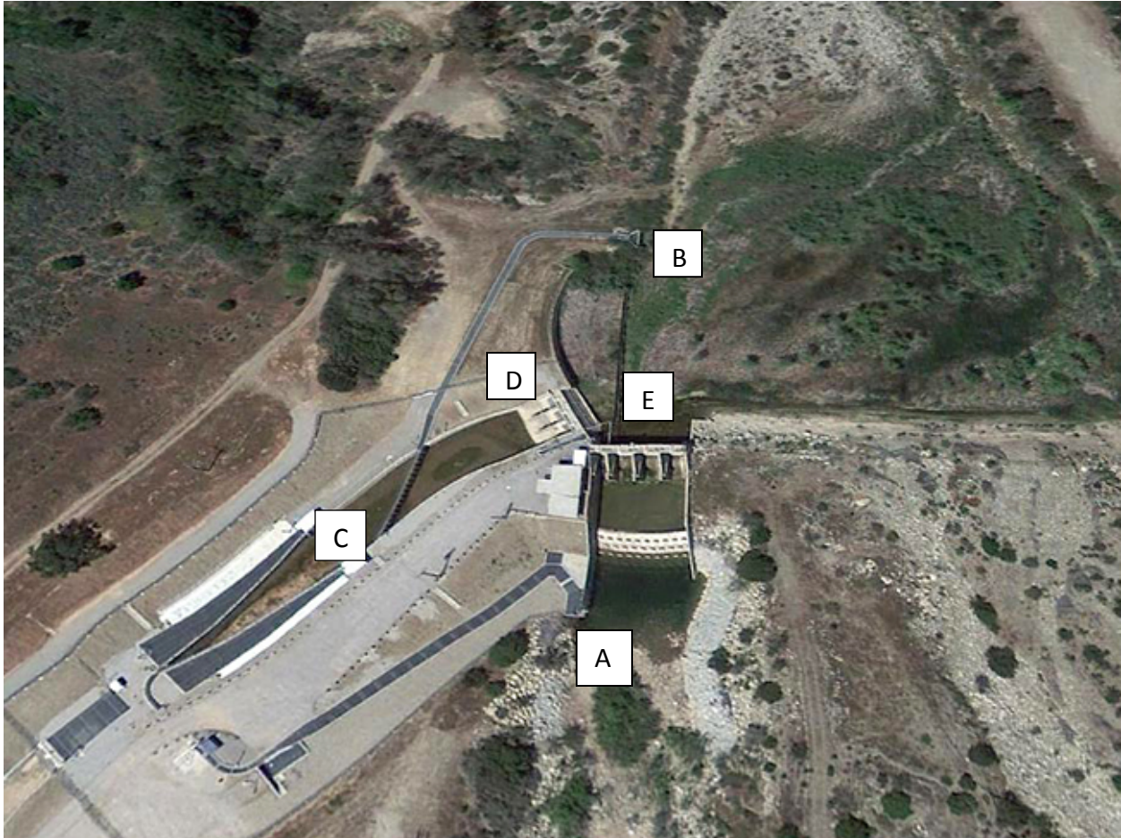
Figure 11. Robles Diversion Fish Passage Facilities, Ventura River. A - Fish ladder entrance. B - Fish ladder exit. C - Diversion fish screens. D - Diversion intake. E - High-flow bypass.
