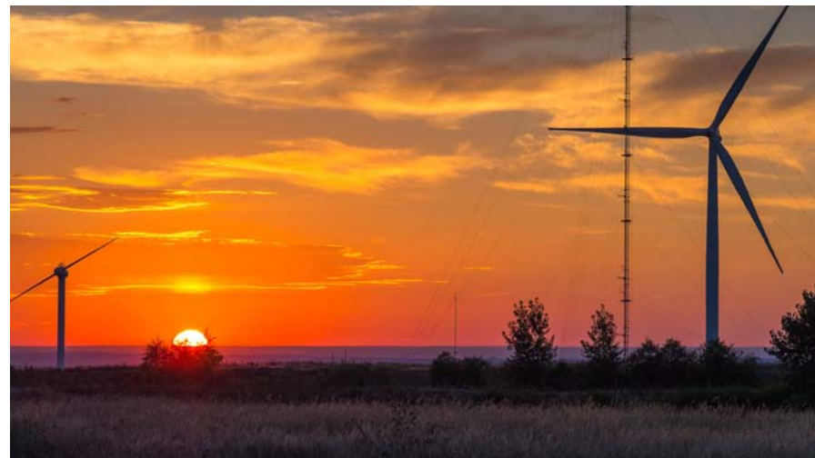
Turbines at the National Renewable Energy Laboratory's National Wind Technology Center. Photo credit: Will von Dauster/NOAA
