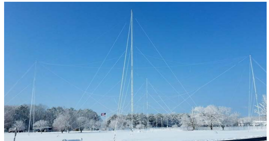
The log periodic transmitting antenna at Wallops Island, Virginia, after an unusual late spring snowstorm. The antenna is 250x250 ft square, 120 ft tall and contains a mile of wire. It is normally not possible to photograph the complexity of the wires in this antenna because they are difficult to see at distances large enough to capture the entire antenna.
