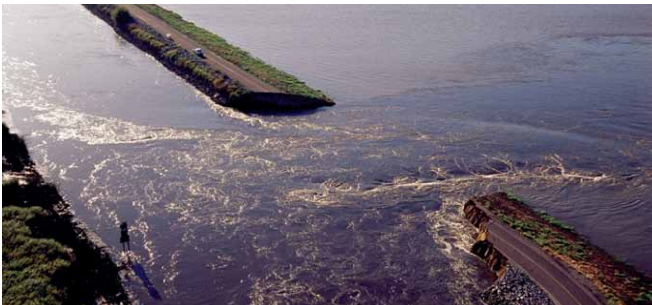
A broken California levee in 2004.
