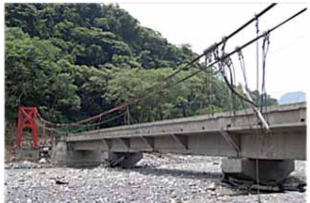
This bridge over the Peikang River has been partly buried as a result of earthquake- and typhoon-triggered landslides, which fed massive volumes of sediment to the river following the 1999 Chichi earthquake.
