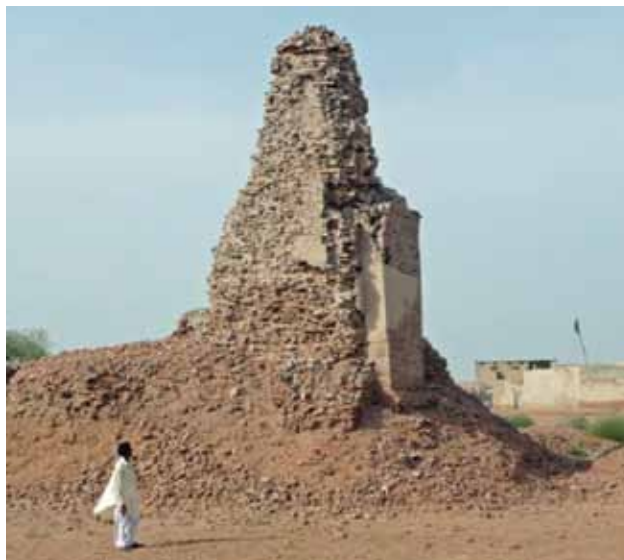
The “Thul” at Mansurah in 2008. This masonry tower is all that remains of fortified town of Mansurah, the ancient capital of Sindh province that was destroyed by an earthquake c. 980 AD. In 19th century archaeological excavations, skeletons were found crushed by bricks. Recent excavations revealed four massive bronze door knockers buried deep beneath the ruins of the largest building, objects that had escaped looting in the past millennium, which would surely have been removed if the city had, instead of being shaken by an earthquake, been sacked by an invading army.
