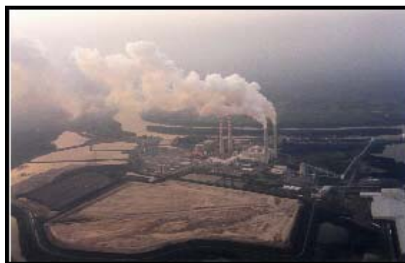
Large power plant located in Tennessee.
