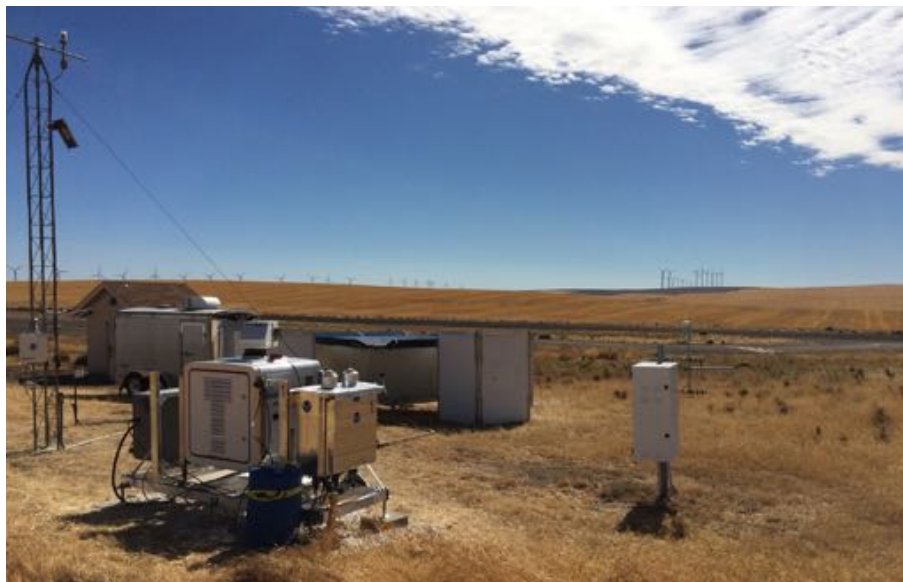
NOAA Doppler wind lidar (in foreground) deployed during WFIP2 near a wind farm along the Columbia River. Photo: Aditya Choukulkar/CIRES
