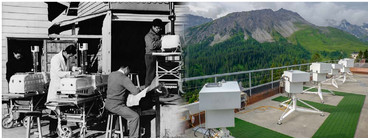
Figure 1 - Continuous Total Ozone Measurements (from manual operations to automatic instrumentation– from the 1950s to today)
