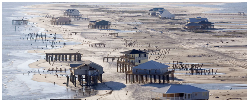
Top: Hurricane Katrina on August 28, 2005 as it approached New Orleans. Middle and bottom images show Katrina's damage along the Louisiana and Mississippi coasts.
