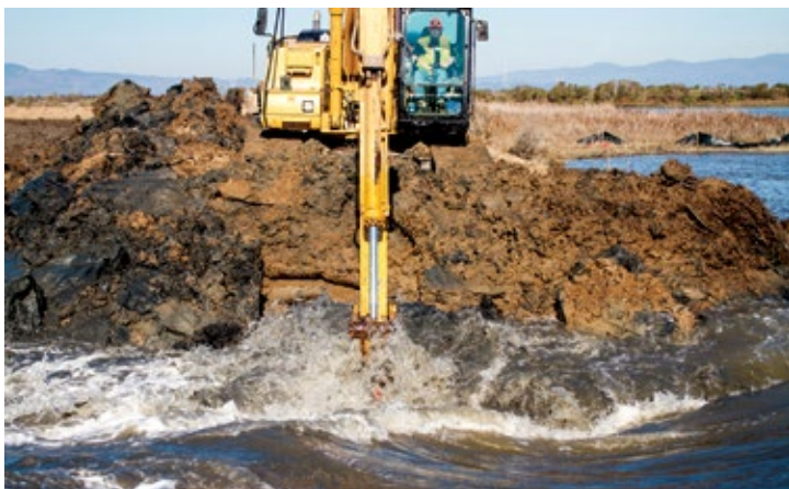
Water gushes through the breach to create wetland habitat at San Pablo Bay Refuge.
