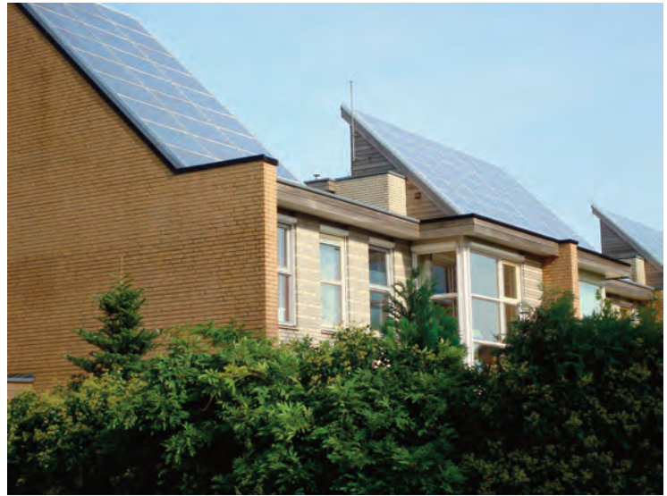
Roof-top Solar Collectors for Residences in Amersfoort, Holland
