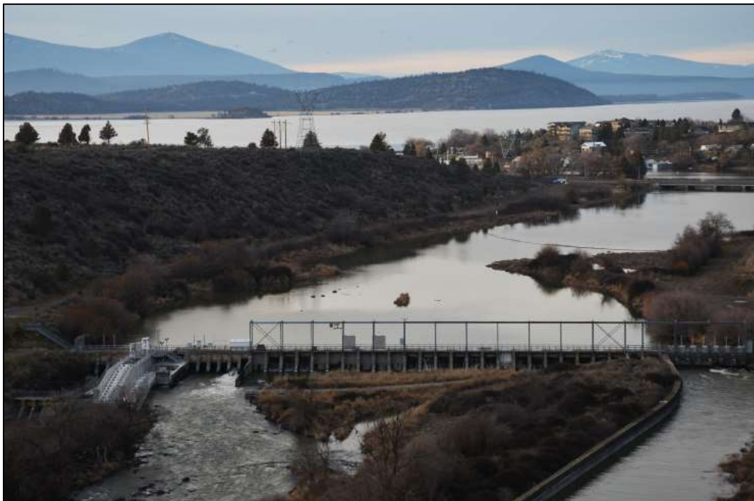
Figure 5–2. Link River Dam, at the outlet of Upper Klamath Lake.
