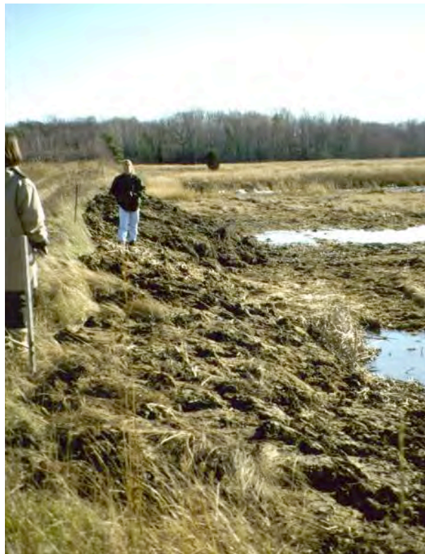
Figure 6. Exposed soils on salt marsh fill.
