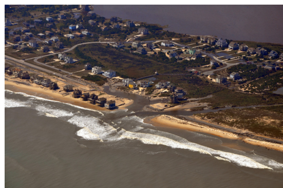
Flooding from Hurricane Irene in August, 2011 sliced through Highway 12 on the Outer Banks of North Carolina. Photo by The Program for the Study of Developed Shorelines, http://psds.wcu.edu
