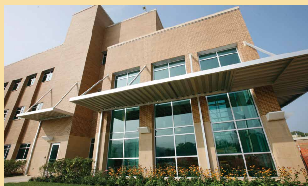
BESC Headquarters. ORNL’s Joint Institute for Biological Sciences facility in Oak Ridge, Tennessee, houses BESC administration and ORNL-based research staff. [Image courtesy Oak Ridge National Laboratory]
