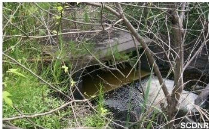
Storm water outfall
