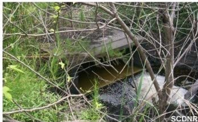
Storm water outfall
