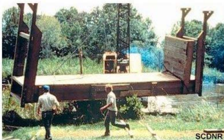
Impoundment trunk being installed
