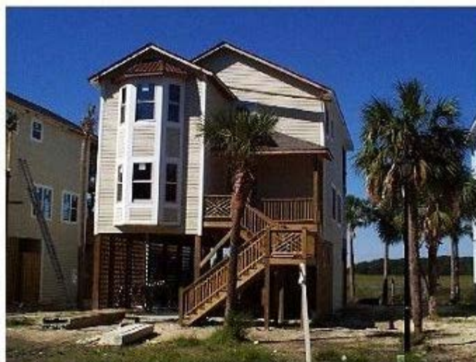
New construction on Edisto Beach
