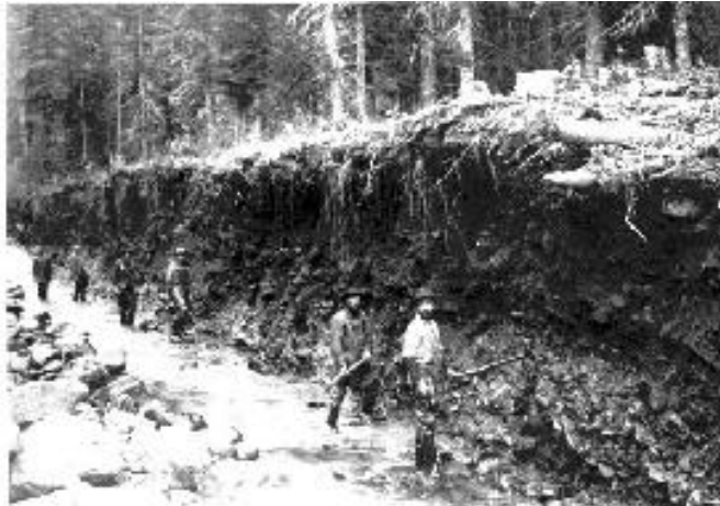
Figure 2-8. Typical Legacy Mining of Placer Deposits in East Eagle Creek (Coeur d'Alene basin), circa 1860s
