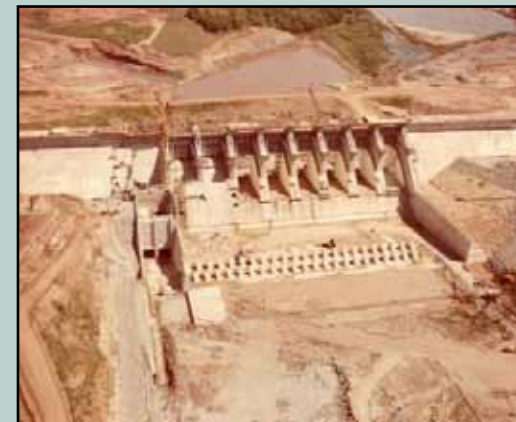
Kaw Lake Dam under construction
