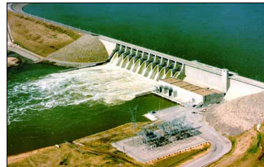
Lake Eufaula dam and powerhouse is one of the 18 hydropower facilities in the Southwestern Division. Lake Eufaula is located in the eastern part of Oklahoma on the Canadian River. (File photo)
