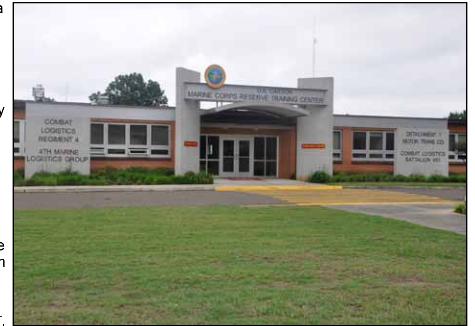
The Fort Worth District Energy Audits and Assessments team conducted a May 28 energy audit at the D.A Carson Marine Corps Reserve Training Center, in Texarkana, Texas. Once the audit is complete, the Corps will provide the Marine Corps Reserve unit an assessment on how they can become more energy efficient. (Photo by Fort Worth District)
