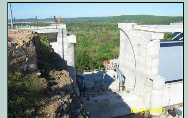
Tenkiller Auxiliary Spillway construction
