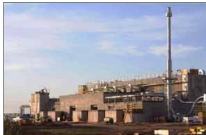
High Explosive Pressing Facility at 95 percent complete.
