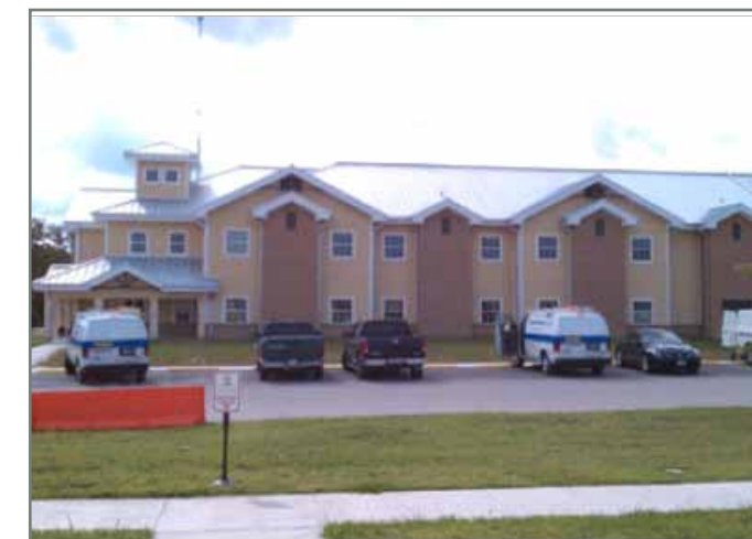
Temple VA Long Term Care Facility, Temple, Texas
