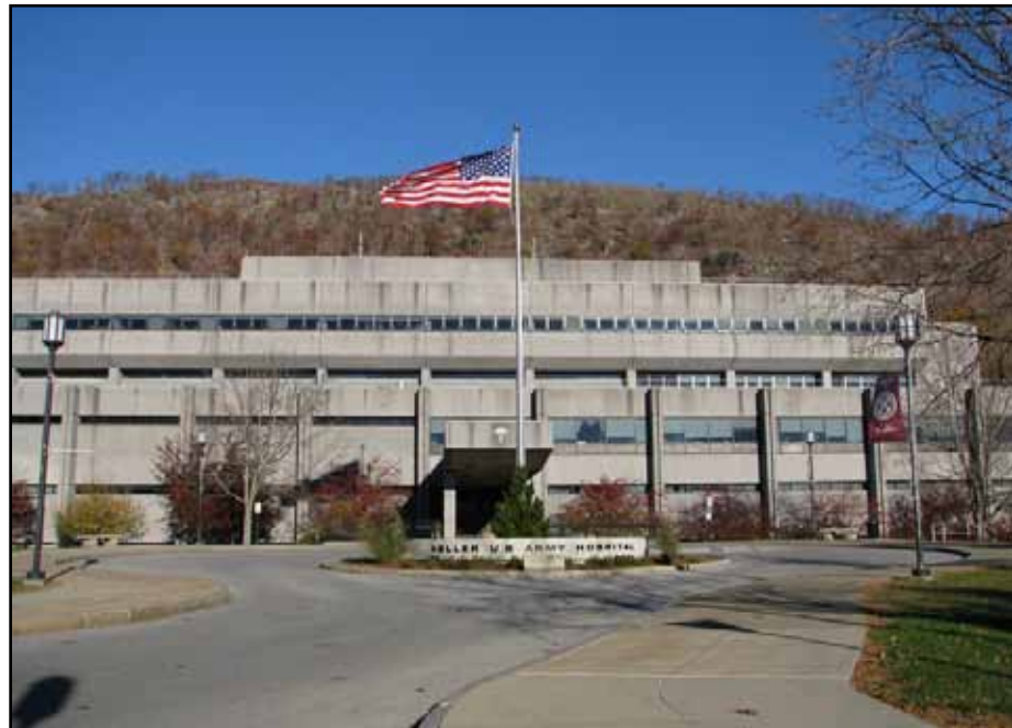
Keller Army Community Hospital renewal project at West Point, N.Y. (Courtesy photo)
