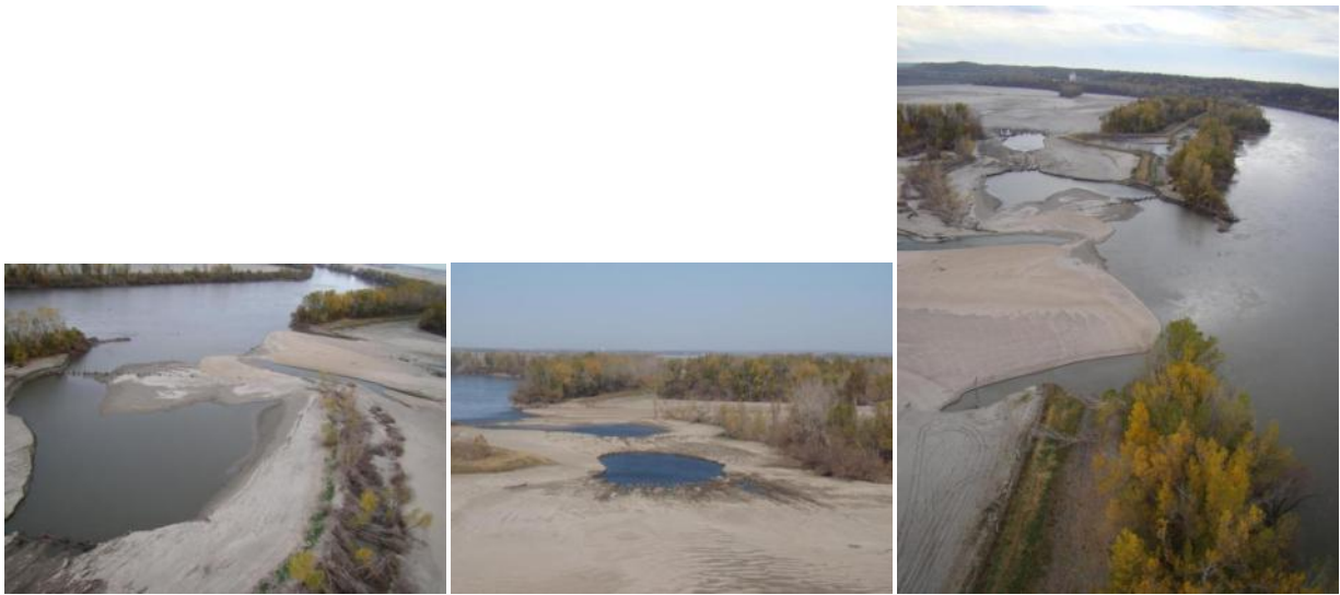
Figure 4-4(d): Aerial Photos of Flood Damage Submitted by Mr. Derks
