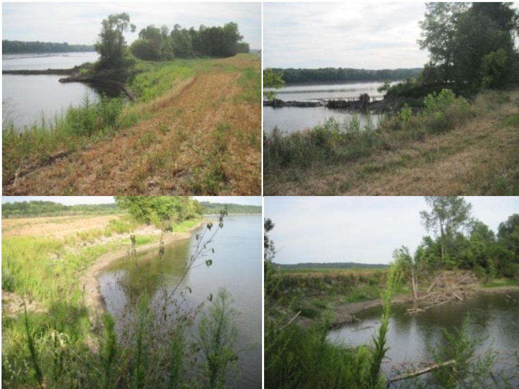
Figure 2-19(a): Submitted Photos of Area of Concern between RM 163 and RM 164
