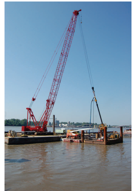
Drilling Angled Piles for Stringout—St Louis District
