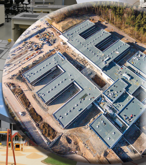
Elements of the new Stuttgart elementary and high-school campus (U.S. Army photos by Chris Augsburger)
