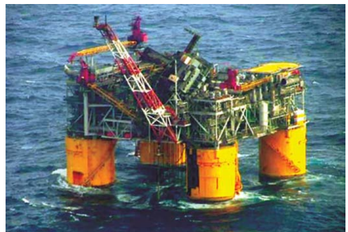
Figure 20. Damaged offshore platform after Hurricane Katrina
