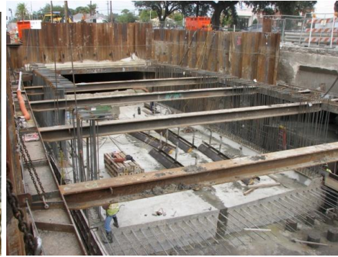
4. Box culvert construction takes place
