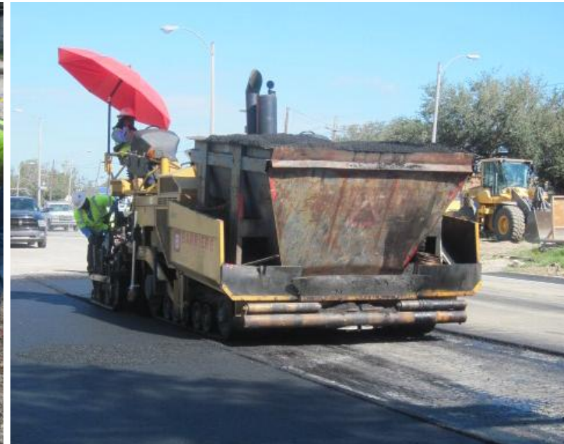
6. Roadway is restored
