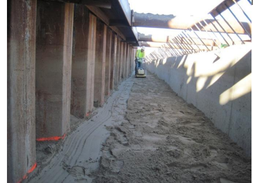
5. Materials are backfilled into the ground
