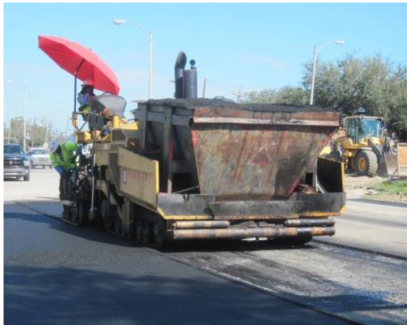
6. Roadway is restored
