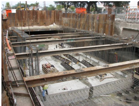
4. Box culvert construction takes place
