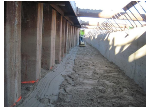
5. Materials are backfilled into the ground
