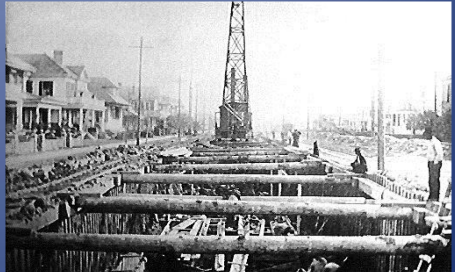
Napoleon Avenue Canal Construction, 1912 ( http://nutrias.org/photos/ )
