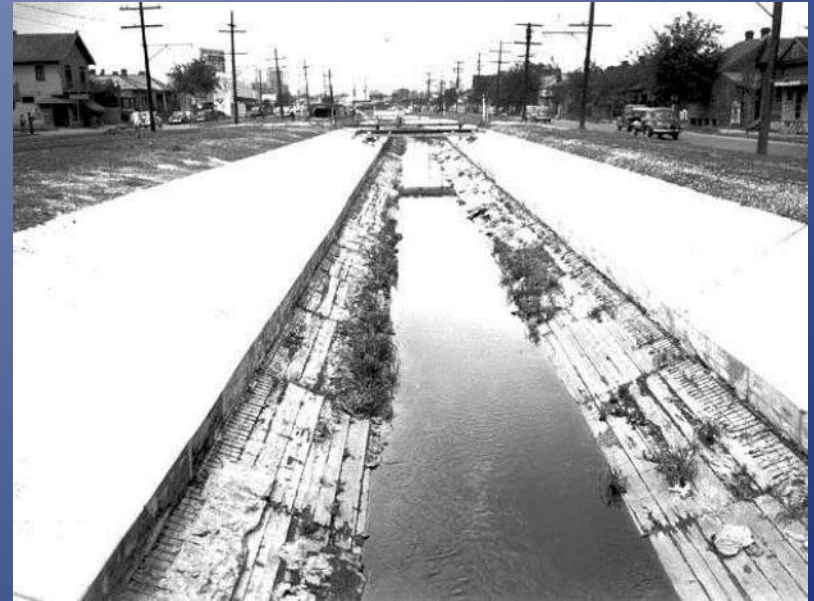
South Claiborne Canal after 1940s Improvements ( http://nutrias.org/photos/wpa/wpa15.htm )
