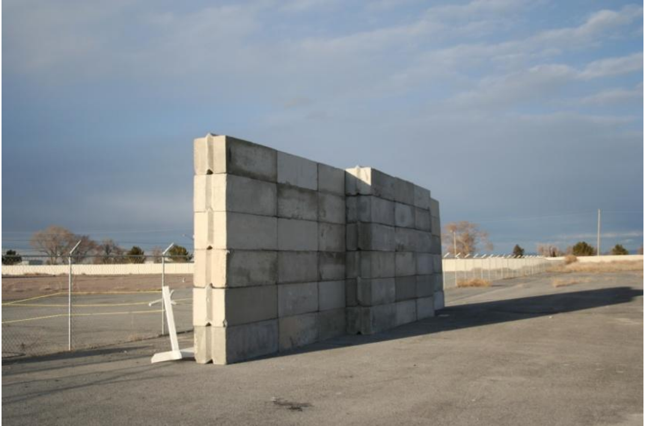
Figure A-5. Example of beam stop assembled using concrete blocks; this picture shows a typical beam stop for the Varitron-III shielding. Each block is 2 ft. thick, 2 ft. tall and 6 ft. long. The delivery and assembly of shield blocks requires semi trucks and forklifts; the movement of a large number of blocks usually only happens once every few years. For example, shield blocks could be placed in front of a trailer or control station pad, along the sides of the linac support building for uncollimated operations or so work could be conducted within the building, to prevent the beam from traveling outside the linac support building fenced area (see Figure A-3), or placed along the down range road to stop the beam from leaving the fenced portion of the SOX Range. This allows work with shorter beam lines, reducing the size of the radiologically control footprint or area.
