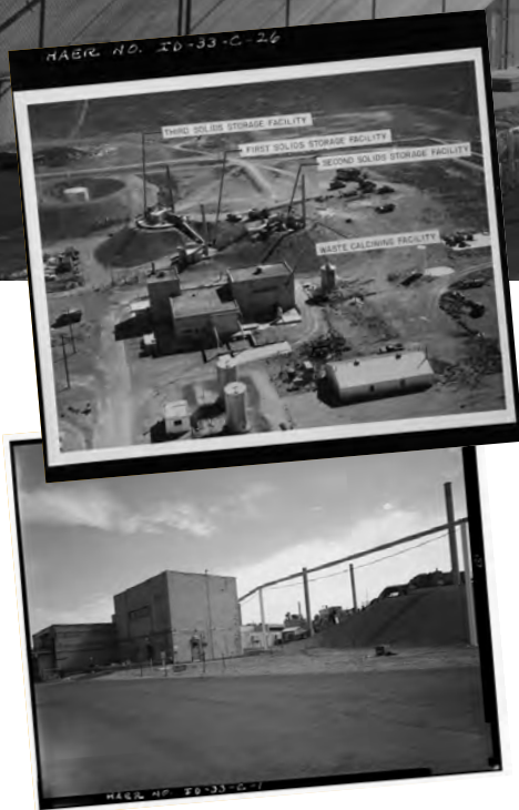
(Left) Historic American Engineering Record Photography of Old Waste Calcining Plant Taken Prior to Demolition. Source: Library of Congress.
