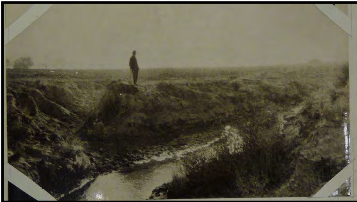
Figure 27: View of Mason Drain Below the Purdum junction (NMID110)
