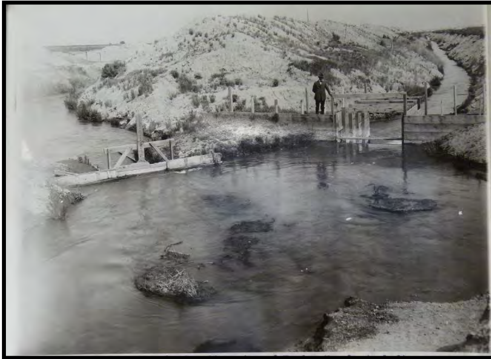
Figure 26: View of Wilson Drain showing Diversion of Feeder No. 1 on left, June 5, 1919 (NMID108)
