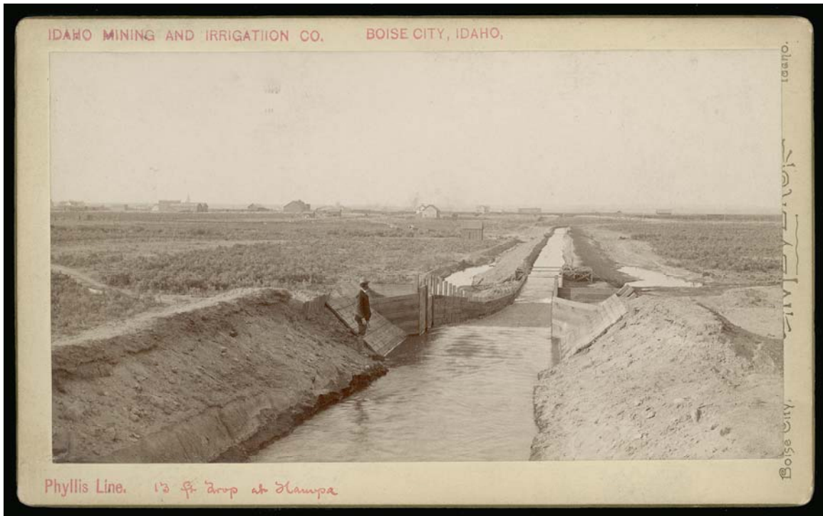
Figure 2 Phyllis Line, 13-foot Drop at Nampa, c. 1890 Courtesy of Brigham Young University, Idaho Mining and Irrigation Co. Photo Collection
