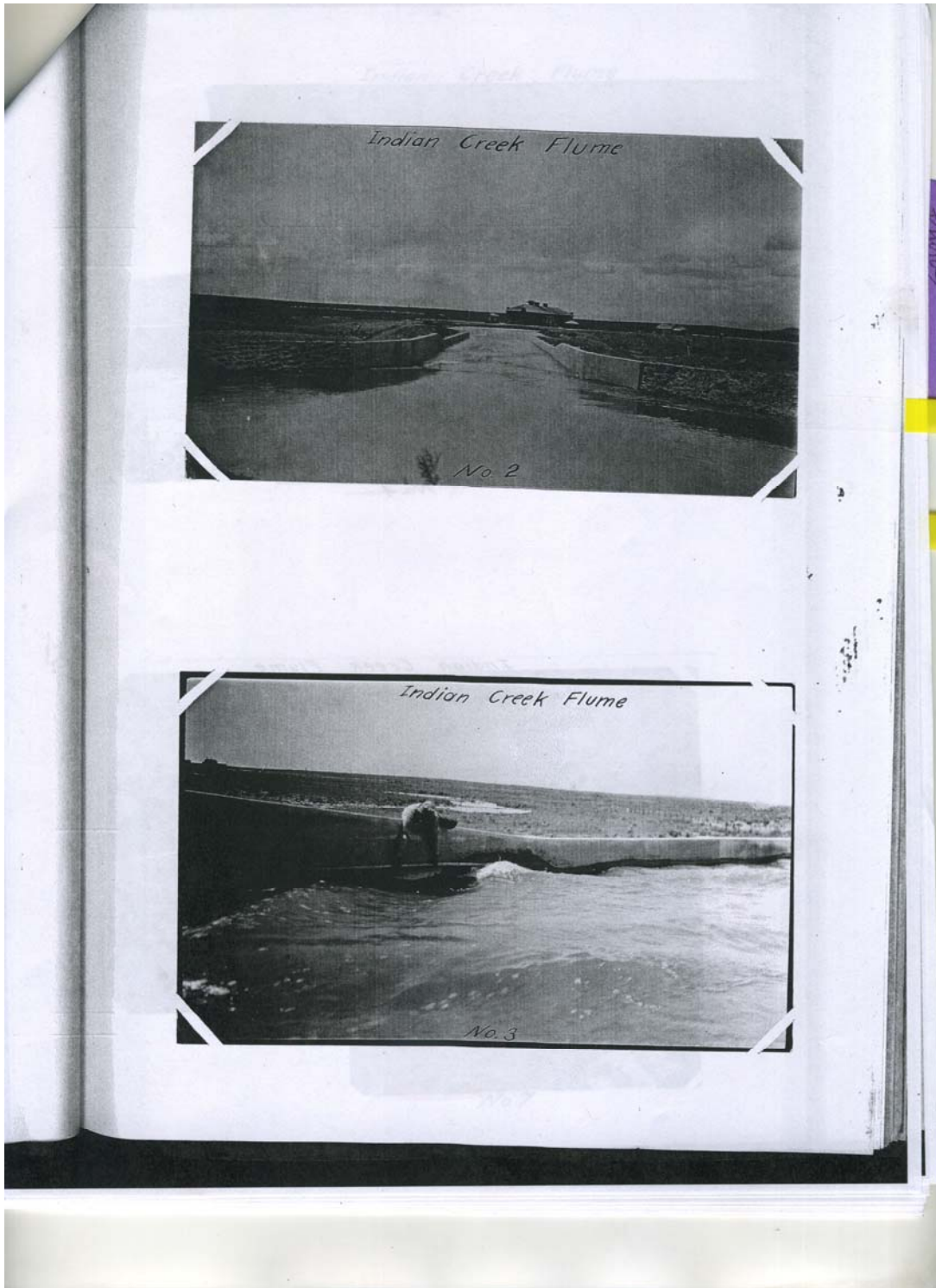
Figure 29 Indian Creek Flume 123
