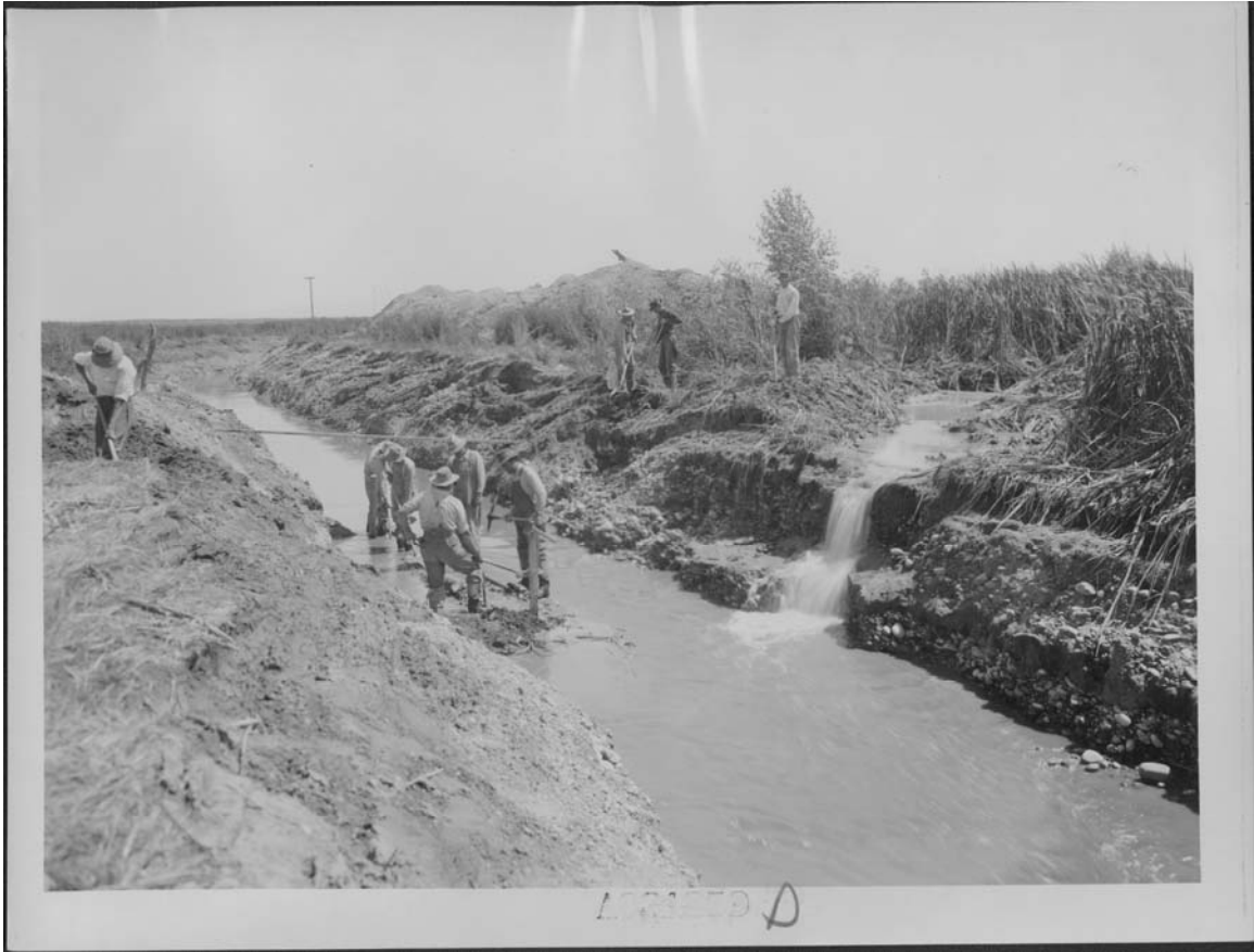
Figure 24 June 22, 1914 "Excavating for bridge sills on road crossing on Purdam Drain." 110
