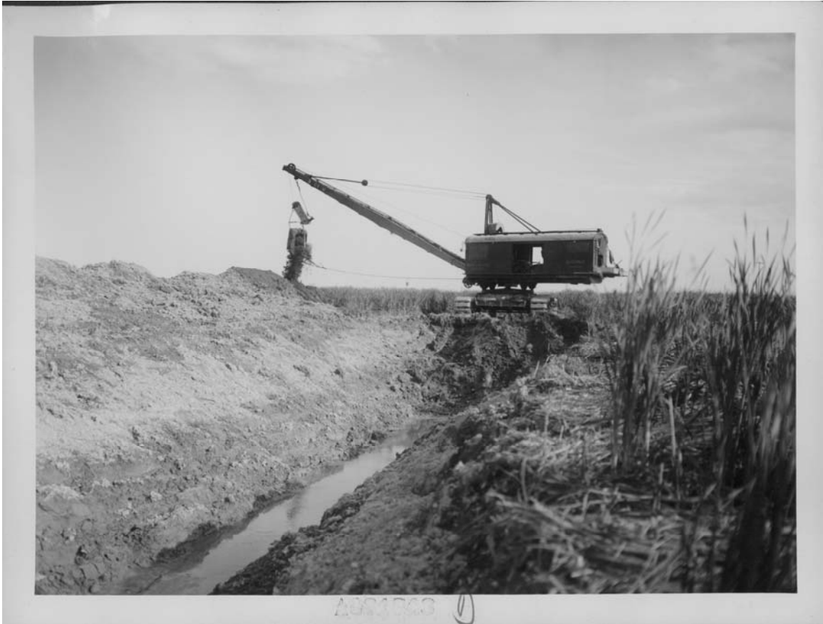
Figure 15 June 22, 1914 "Electric Dredge on Wilson Slough Drain." 101
