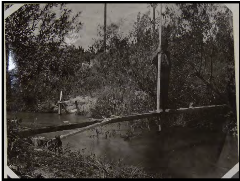
Figure 25: Photograph of Construction of Bridge over Indian Creek, No Date (NMID105)
