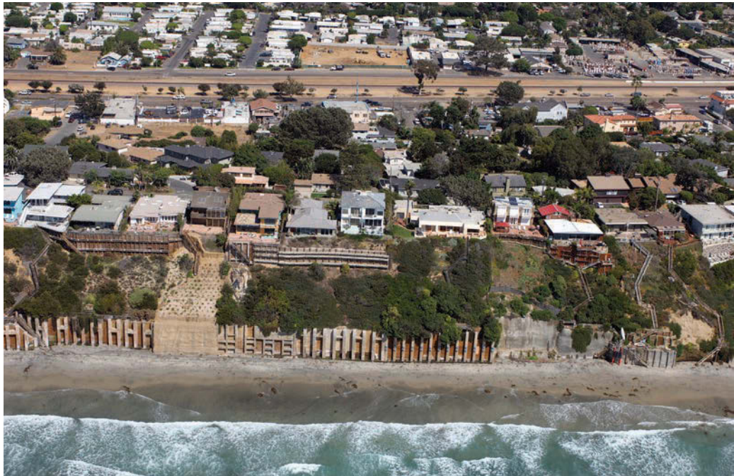
Figure 9.8 Coastal armoring in Southern California. One-third of the shoreline of Southern California (including Ventura, Los Angeles, Orange and San Diego Counties) has now been armored. The photo shows the shoreline in 2010 in Encinitas, in northern San Diego County. Photo courtesy of Kenneth and Gabrielle Adelman of the California Coastal Records Project ( http://www.californiacoastline.org/ ).
