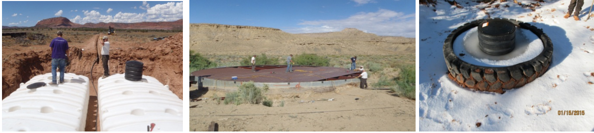
Left, installing storage tanks for wildlife drinker at Eightmile; center, putting a lid on the Coyote storage tank. Lid have drastically reduced mortalities at GSENM waters. Right, new Brown Springs trough installed outside riparian area. Riparian area will be fenced in 2015.
