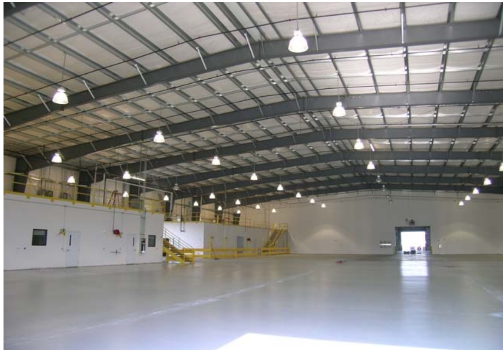
Interior Selma Prefabricated Building
