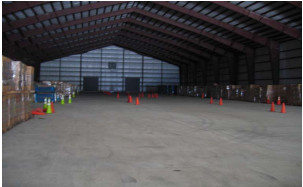
Interior Cumberland Prefabricated Building
