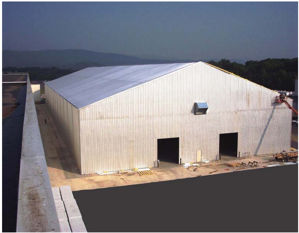
Exterior Cumberland Prefabricated Building
