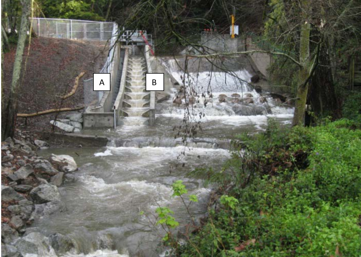
Figure. 6. Fish Passage Facilities, Corralitos Creek, Pajaro River. Photo courtesy Kittleson Environmental Consulting. A – Juvenile fish passage. B – Adult fish passage.
