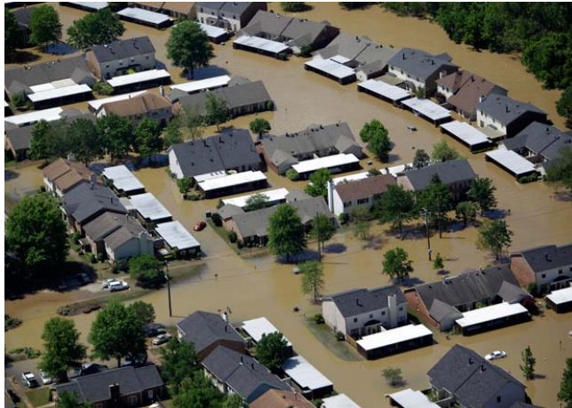
Figure 2. Nashville flooding, FEMA Disaster No. DR 1909 TN (Source: FEMA)
