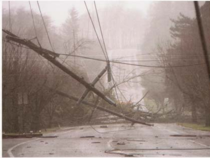
Figure 4. Dangerous debris situation (Source: FEMA)
