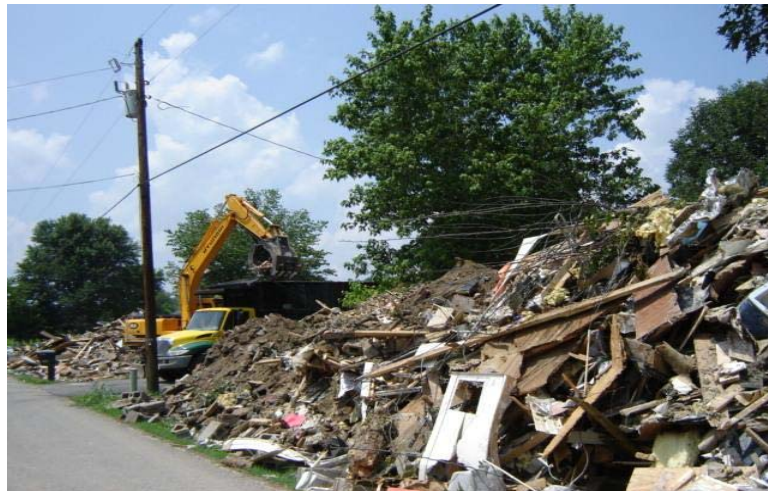
Figure 1. Nashville flooding, FEMA Disaster No. DR 1909 TN (Source: FEMA)
