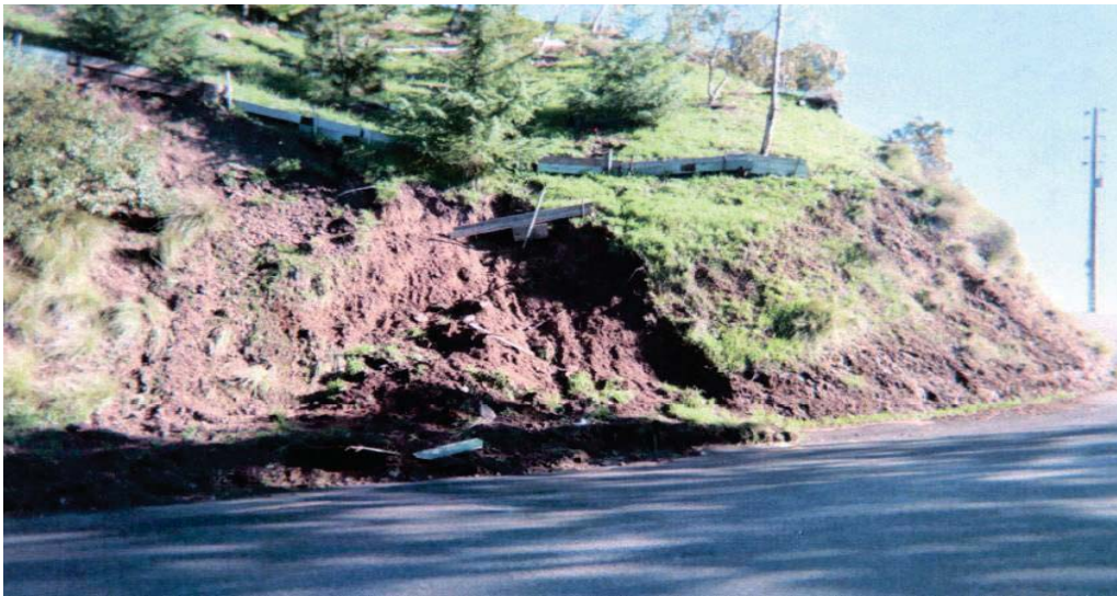
Figure 1: Debris Removal: Roads, Shoulders, and Drains Source: FEMA Project Worksheet 2940.
