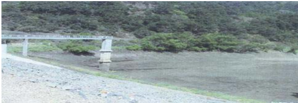
Figure 3: Debris Basin Post-Cleanout (June 7, 2005) (Little Dalton) Source: FEMA Project Worksheet 2275.
