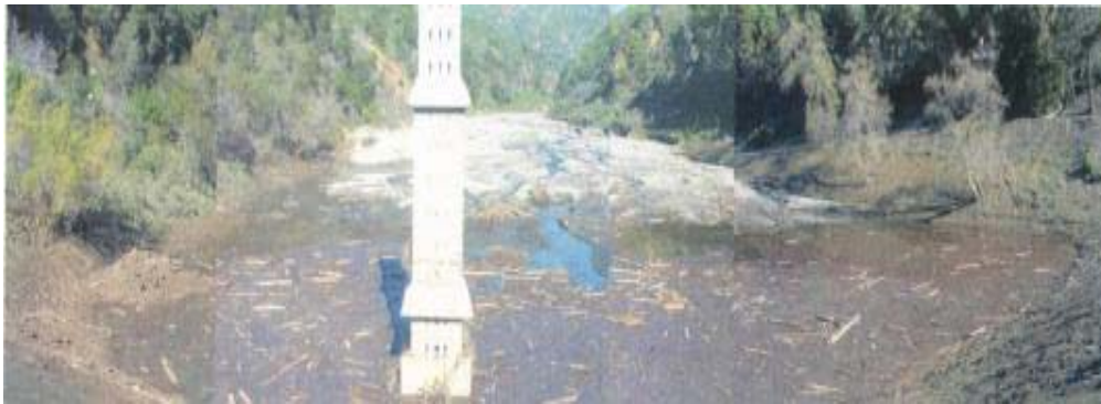
Figure 2: Debris Basin Pre-Storm (January 19, 2005) (Little Dalton) Source: FEMA Project Worksheet 2275.
