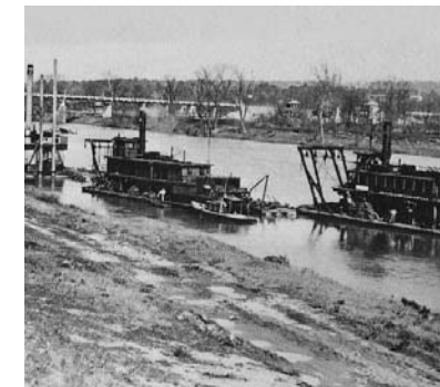
Two Corps snagboats and a dredge clear the Savannah River at Augusta, Ga., in the 1920s.
