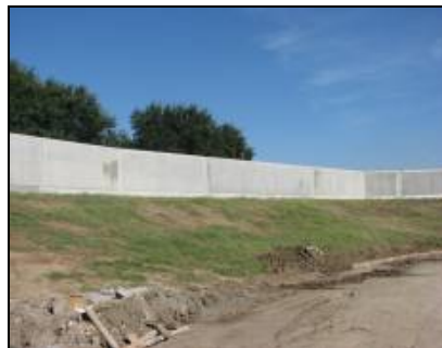
Floodwall near Bayou St. John
