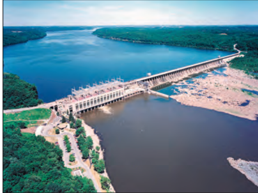
Photograph of Conowingo Dam, courtesy of Exelon Corp.
