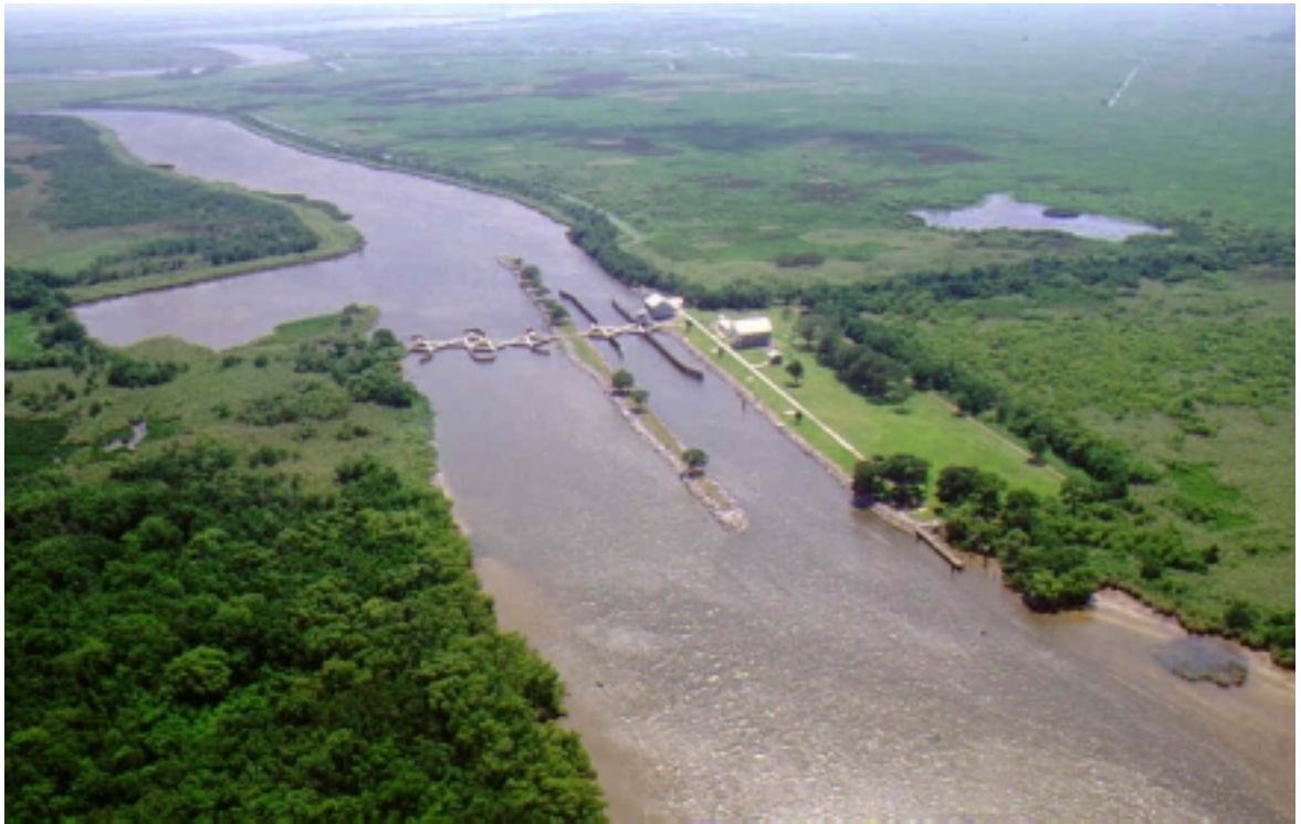
Catfish Point Control Structure
