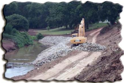
Rock is placed to prevent further erosion.
