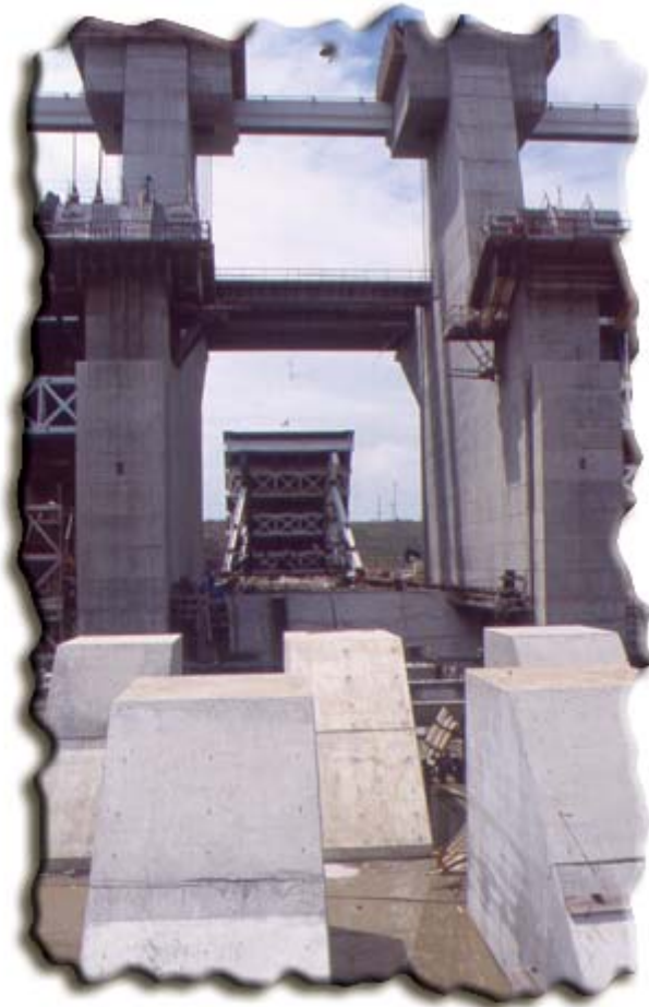
Final gate installation at the Old River Control Auxiliary Structure, April 1985.
