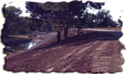
The bayou's banks are cleared and graded.
