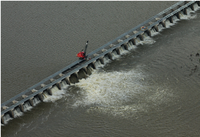
Map of Bonnet Carré Spillway (top), and aerial of the spillway in operation during the flood of 2011 (bottom).
