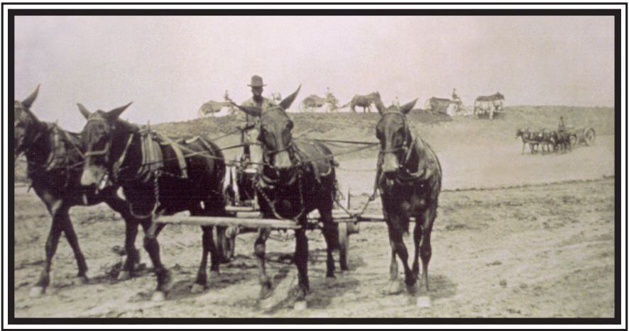
Early levee construction
