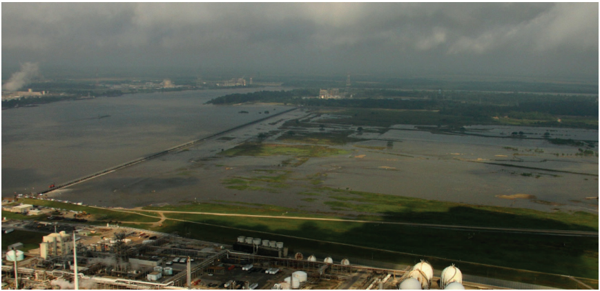
High altitude view of the spillway (center) stretching from the Mississippi River to Lake Pontchartrain, looking upriver. This photo was taken just after the first bays were opened during the flood of 2011.
