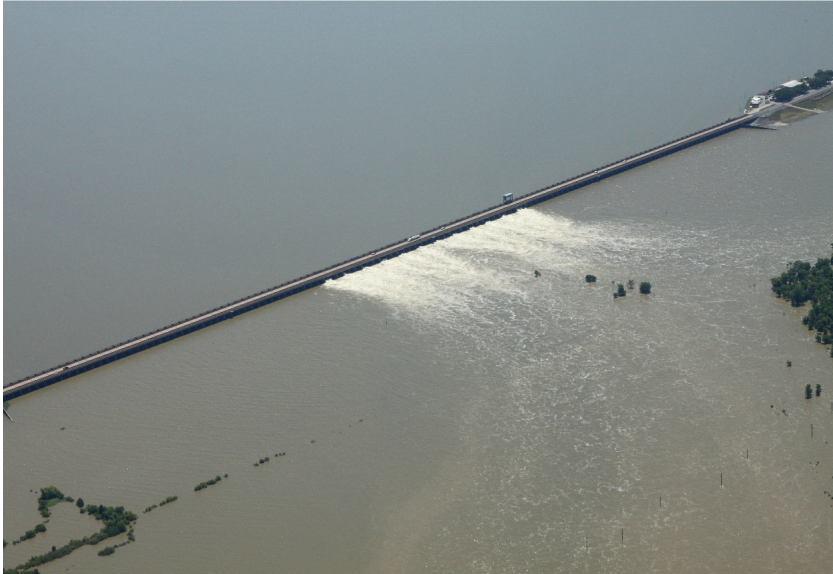
The Corps operated the Morganza Floodway for only the second time ever (and the first time for its intended purpose) in 2011 to divert excess Mississippi River water to the Atchafalaya River Basin and relieve pressure on the mainline Mississippi River levees.
