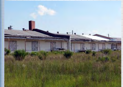
Fig 5.23 – Some older building create poor visual image
