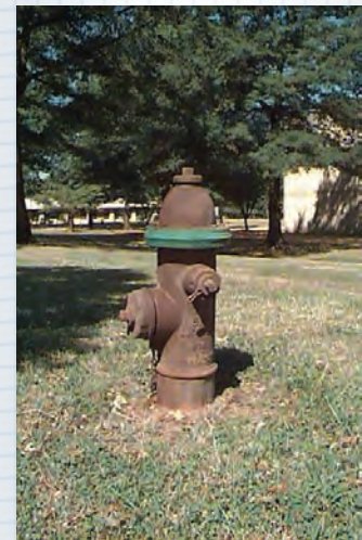
Fig. 11.60 - Fire Hydrants Shall be Nutmeg Brown. Caps Shall Indicate Tested Water Pressure
