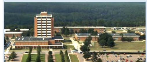
Fig 5.18 – Signal Towers and Academic Facilities comprise the Fort Gordon “Traditional Core” Zone.
