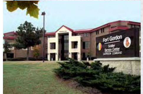
Fig 8.32 – The Darling Hall Material and Color scheme is the model palette for this Visual Zone.
