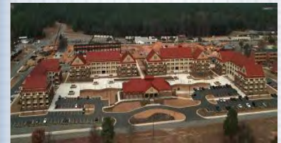
Fig. 3.21 – All Elements of the visual environment should blend to complement one another. (Permanent Party Barracks)
