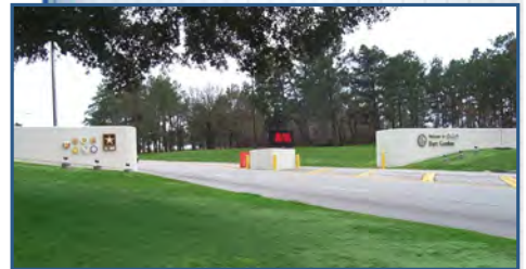
Decorative Wall Beyond Installation Main Gate
