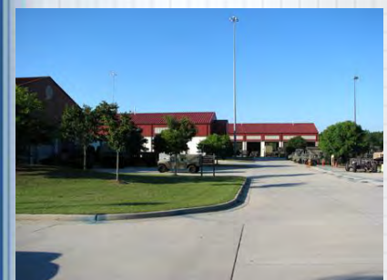
Fig 5.22 – Successful integration of architecture and site
