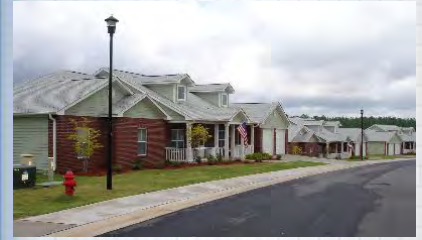
Fig 5.36 – Pedestrian walkways present throughout new housing developments
