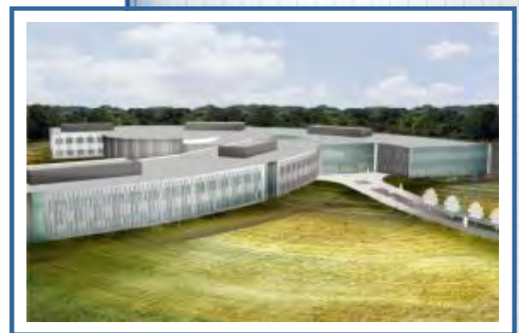
Fig 5.33 – Pre-construction rendering of NSA/CSS GA Operations Center
