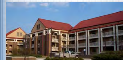
Fig. 3.5 – Similar Exterior Building Materials and Colors Strengthen Installation's Uniform Visual Image
