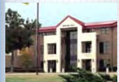
Fig. 8.11 - Entrance at Darling Hall is Well Defined.
