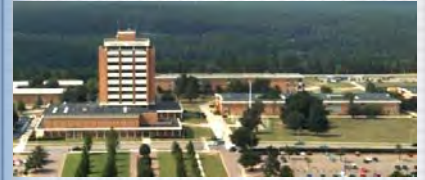
Fig 6.9 – U.S. Army Signal School at Fort Gordon
