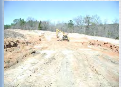
Fig 4.8 – Fort Gordon Borrow Pit
