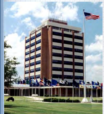
Fig 8.26 – Signal Towers and Instructional Facilities comprise the Fort Gordon “Traditional Core” Zone.
