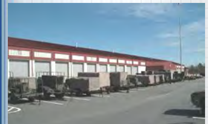
Fig 5.21 – Large industrial buildings are grouped together.
