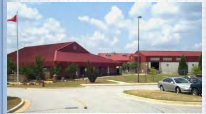
Fig 8.27 – Unified Building exterior colors dominate visual zone – Public Works Admin. Building and Maintenance Facilities – North Industrial Visual Zone
