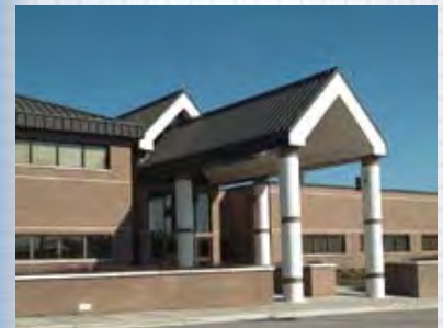
Fig. 8.11 - Prominent Entrance at Reserve Center
