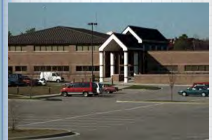
Fig 5.30 – Strong architectural entry features
