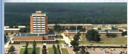
Fig. 3.3 – Fort Gordon Signal Center "Traditional Core"
