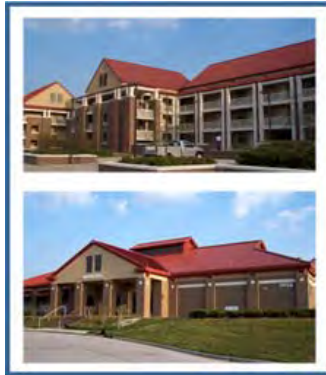
Fig 8.34 – Recently Constructed Facilities within the Zone Offer a Warm Color palette.
