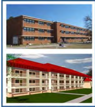
Fig 8.33 – Trainee Barracks Upgrade Program (Currently Under Construction)
