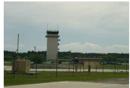
Fig. ES.18 – The tower is utilitarian in design, but architecturally expressive.
