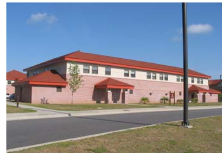
Fig. ES.32 – The exterior materials on Bldg. 1531 include brick, concrete block and stucco walls with metal roof.
