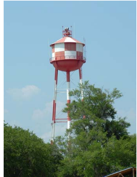
Fig. ES.41 – The historic metal water tower (Bldg. 721) built in 1940.
