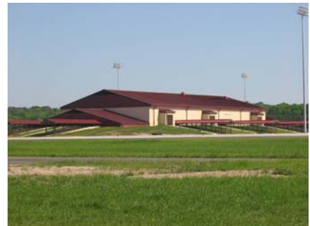
Fig. ES.40 – View of Bldg. 8661 of the Saber Hall complex, which was critical to the SAC ground alert program.
