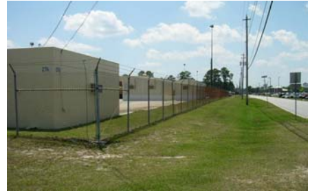
Fig. ES.80 – Fencing provides a reliable barrier to unauthorized entry.
