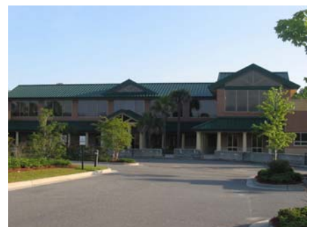
Fig. ES.12 – The entrance to Tuttle Army Health Clinic is architecturally interesting and inviting.
