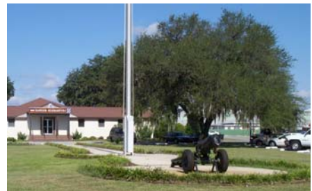
Fig. ES.35 – The Garrison Headquarters was sited to preserve these live oaks.
