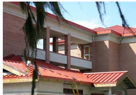
Fig. ES.45 – Example of the uses of materials with integral colors and pre-finished materials in installation standard colors on a new barracks.
