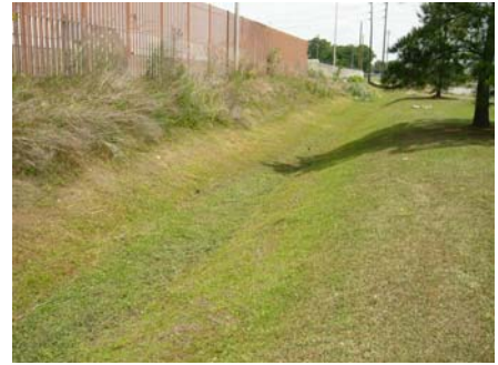
Fig. ES.82 – An earth berm between a road and adjacent building prevents vehicles from approaching the building.
