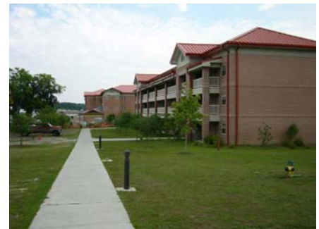
Fig. ES.57 – Walkways promote walking and use of bicycles in place of driving for short trips.
