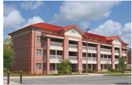
Fig. ES.36 – A typical new barracks (Bldg. 313).
