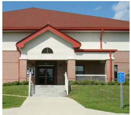
Fig. ES.34 – Portico entrance with masonry columns at a dining facility (Building 110).
