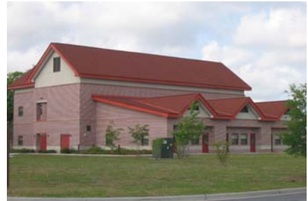
Fig. ES.33 – Small-sized windows, recessed entries and a varying roofline emphasize the human scale of this brigade headquarters (Bldg. 1525).
