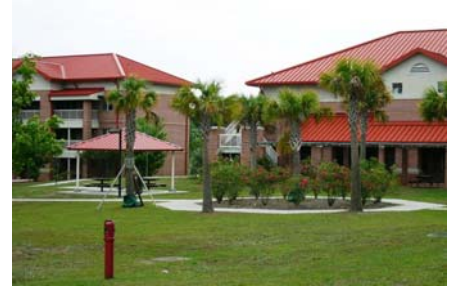
Fig. ES.17 – New planting in the spaces between buildings creates a comfortable and attractive landscape.
