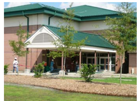
Fig. ES.37 – A portico is a preferred way to emphasize the building entrance.
