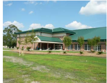
Fig. ES.31 – The Physical Fitness Center exhibits the design characteristics of the Southern Living Station of Choice.
