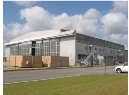
Fig. ES.39 – A 1940–41 hangar (Bldg. 813) in the Flight Line Area of the SAC Operations Historic District.
