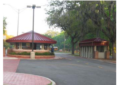
Fig. ES.83 – The Main Gate to Hunter AAF is well-designed for security and appearance.
