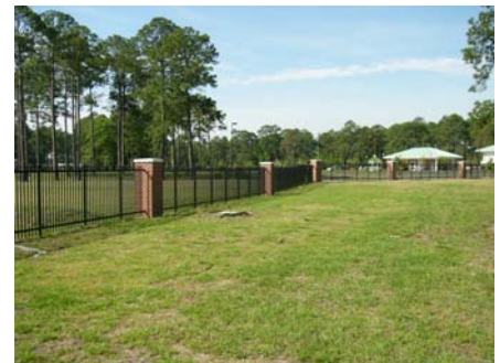
Fig. ES.82 – Perimeter fencing is flanked by cleared areas.
