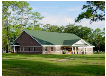
Fig. ES.36 – Front-gabled primary and secondary entrances to the Army Community Service Center (Bldg. 86).
