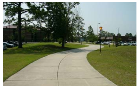
Fig. ES.16 – Walkways connect parking to barracks and adjacent barracks complexes to each other.
