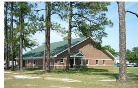
Fig. ES.32 – The Family Readiness Center (Bldg. 87) was sited around existing pine trees.
