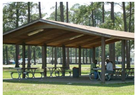
Fig. ES.72 – This attractive shelter provides shade and shelter from rain.
