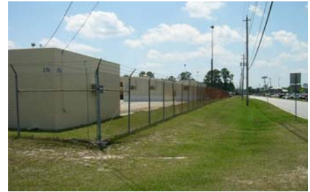
Fig. ES.81 – Fencing provides a reliable barrier to unauthorized entry.
