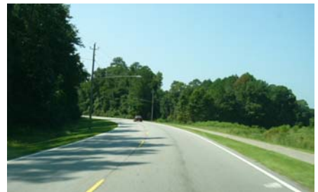
Fig. ES.53 – Hero Road is aligned to blend smoothly with natural features.
