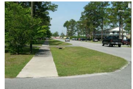
Fig. ES.49 – Hase Road is a secondary roadway.
