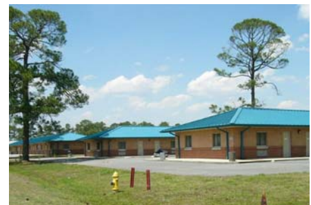
Fig. ES.33 – The Officer/SNCO quarters fit well into the National Guard Visual Zone (Bldgs. 13305 and 13304).
