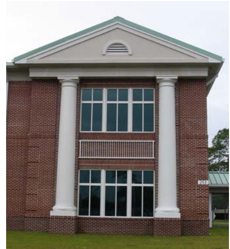
Fig. ES.41 – Detail of the Soldier Service Center (Bldg. 253) that shows typical building materials and colors for the Headquarters Visual Zone.
