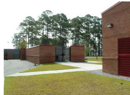
Fig. ES.37 – An example of a well-designed service area enclosure.
