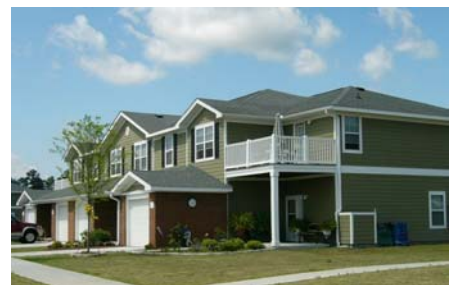
Fig. ES.20 – New housing incorporates architectural detailing to provide visual continuity.
