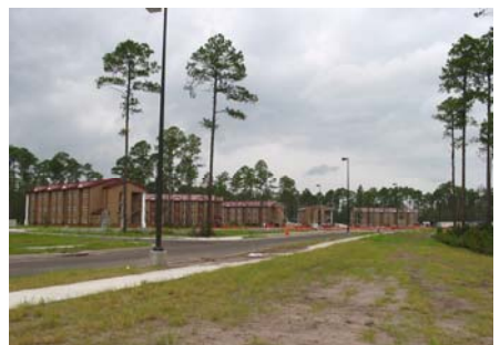
Fig. ES.40 – Green areas surround the barracks in the BCT area.
