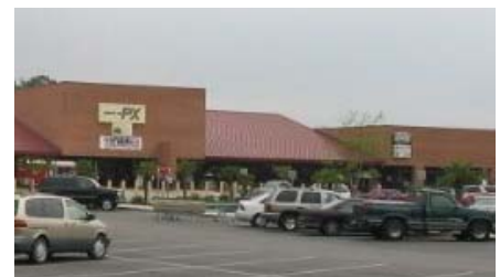
Fig. ES.11 – The entrance to the PX is an attractive and active area.
