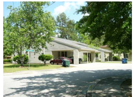
Fig. ES.19 – Short views along streets reduce the scale of the neighborhoods.
