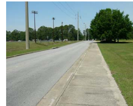
Fig. ES.50 – Sixth Street Extension is a tertiary roadway.
