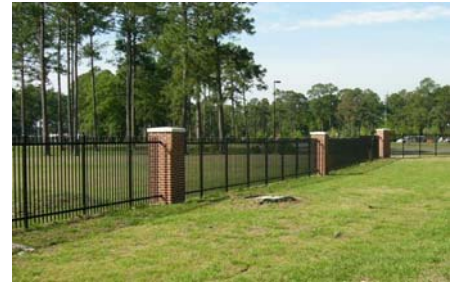
Fig. ES.73 – View of the perimeter fence near the Main Gate.
