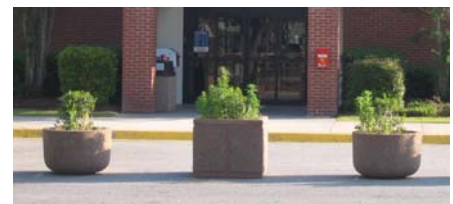
Fig. ES.74 – A concrete barrier planter should be attractive, as well as effective in blocking vehicles.
