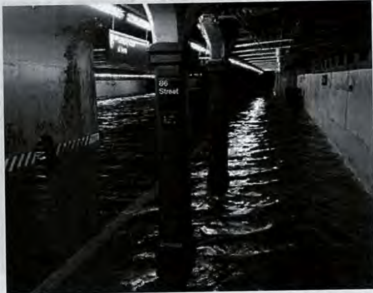
Figure 5.4. The nation's busiest subway system sustained the worst damage in its 108 years of operation on October 29, 2012, as a result of Hurricane Sandy. Millions of people were left without service for at least one week after the storm, as the Metropolitan Transportation Authority rapidly worked to repair extensive flood damage (Photo credit: William Vantuono, Railway Age Magazine , 2012 46 ).
