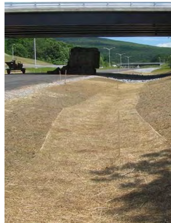
Stormwater swales, Bennington By-Pass.
