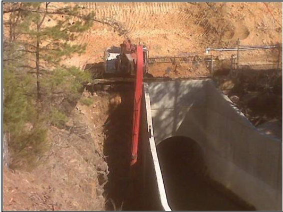
Downstream Filter Construction
