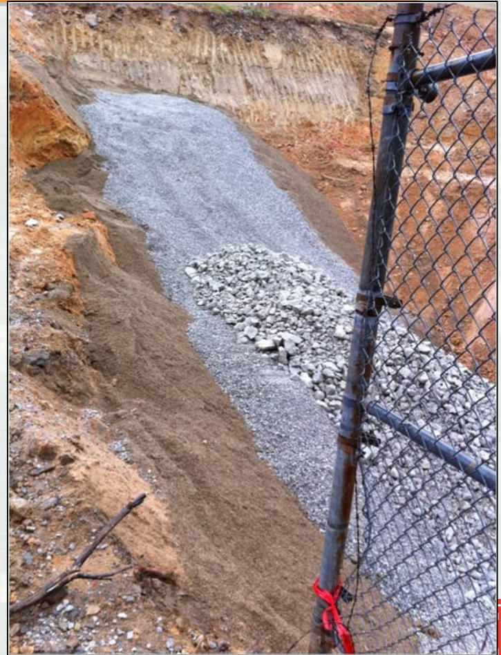
Downstream Filter Construction
