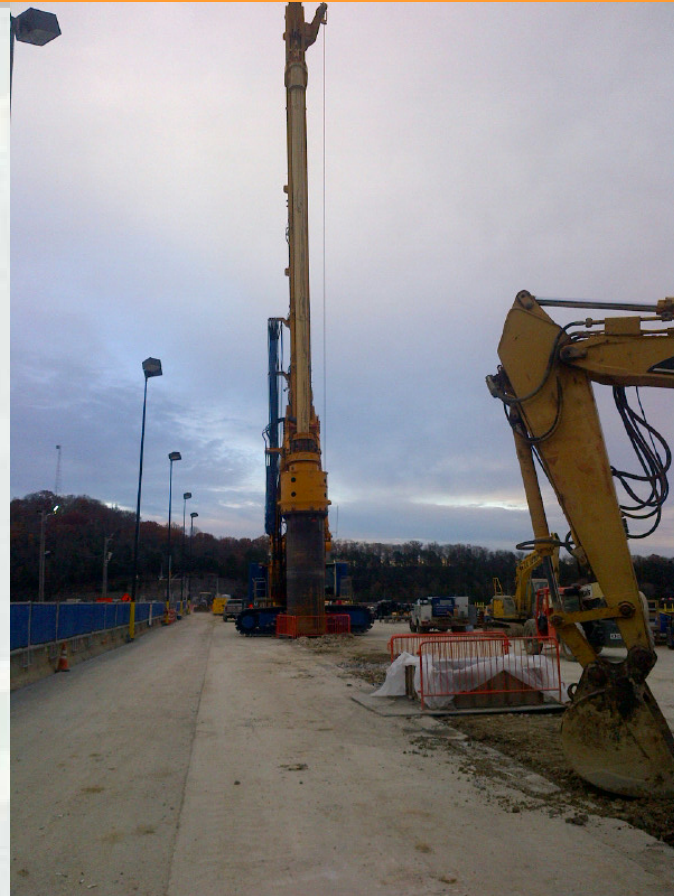
Chimney Filter Construction
