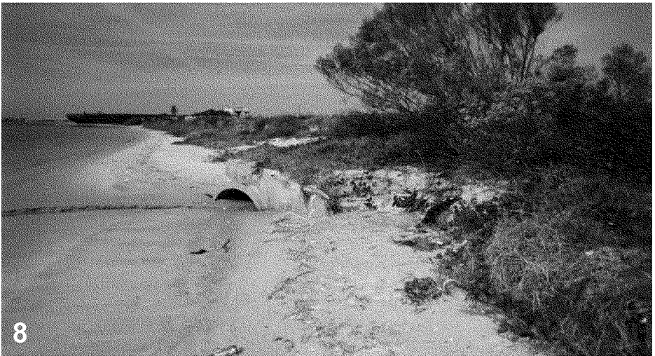
36-inch Stormwater Outlet (East of WTB)
