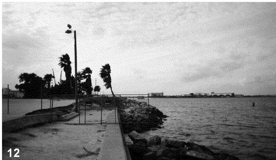
Seawall Along South Side of Channel (Adjacent to WTB Area)
