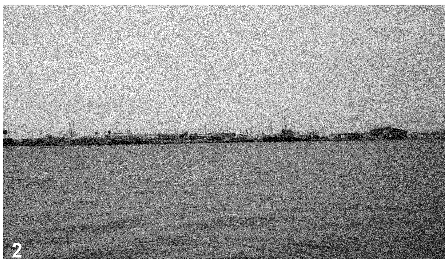
South Side of Channel at WTB Area
