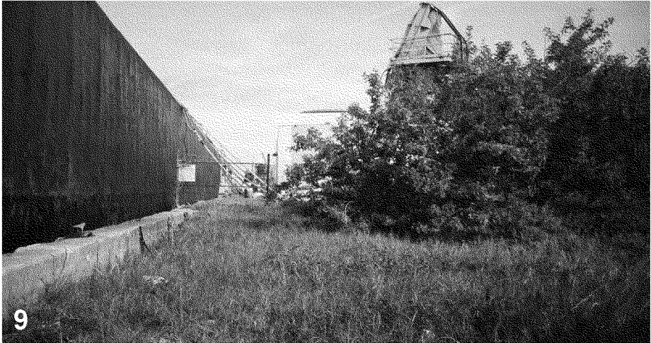
Seawall Along East Side of WTB (Beyel Brother, Inc. Lease)
