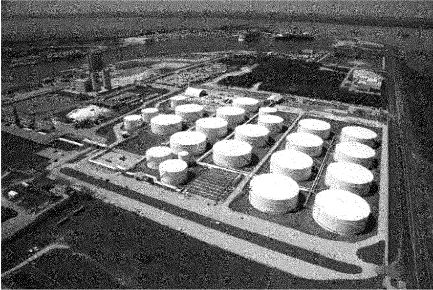
Figure 2-1 Seaport Canaveral Fuel Terminal
