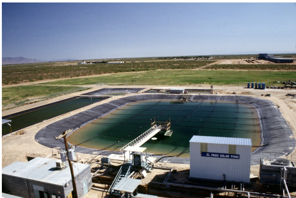
Figure A21. Solar pond test facility at the University of Texas El Paso. Photo by NREL 08841
