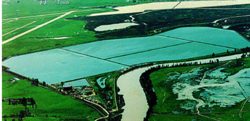
Figure A23. Typical oxidation pond. 93
