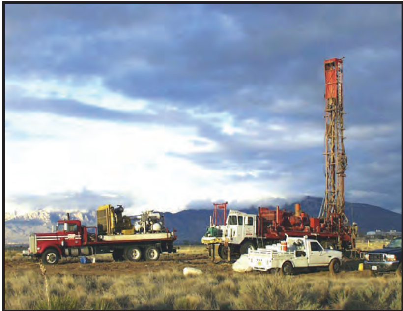
Mixed Waste Landfill Drilling Operations
