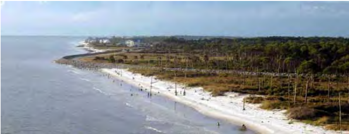
Figure 7.1. A road initially built inland of a receding shoreline is now in the sea. Stump Hole area of Cape San Blas, Florida (2005 FDOT photo)
