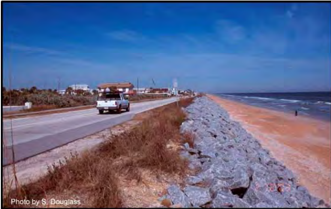
Figure 6.7. Seawall protecting a coastal highway. Florida Highway A1A, Flagler Beach, FL
