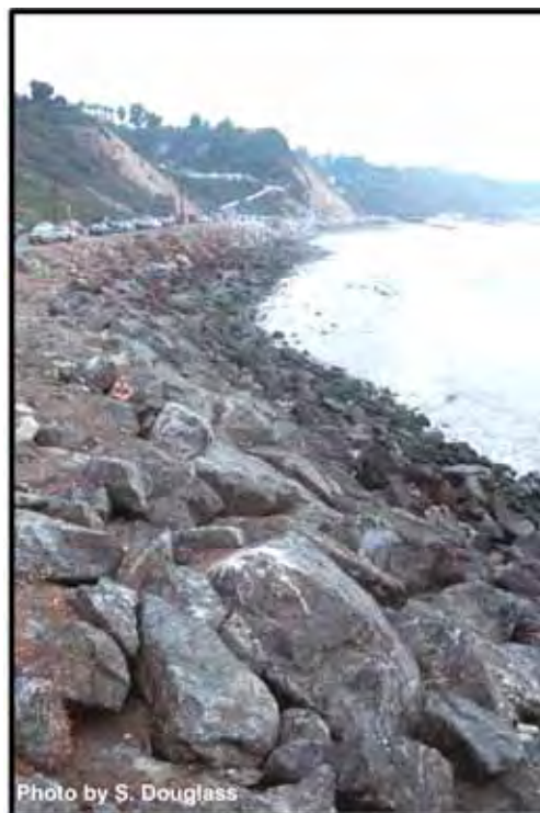
Figure 6.6. Seawall protecting a coastal highway. Pacific Coast Highway, Pacific Palisades, California (2003)
