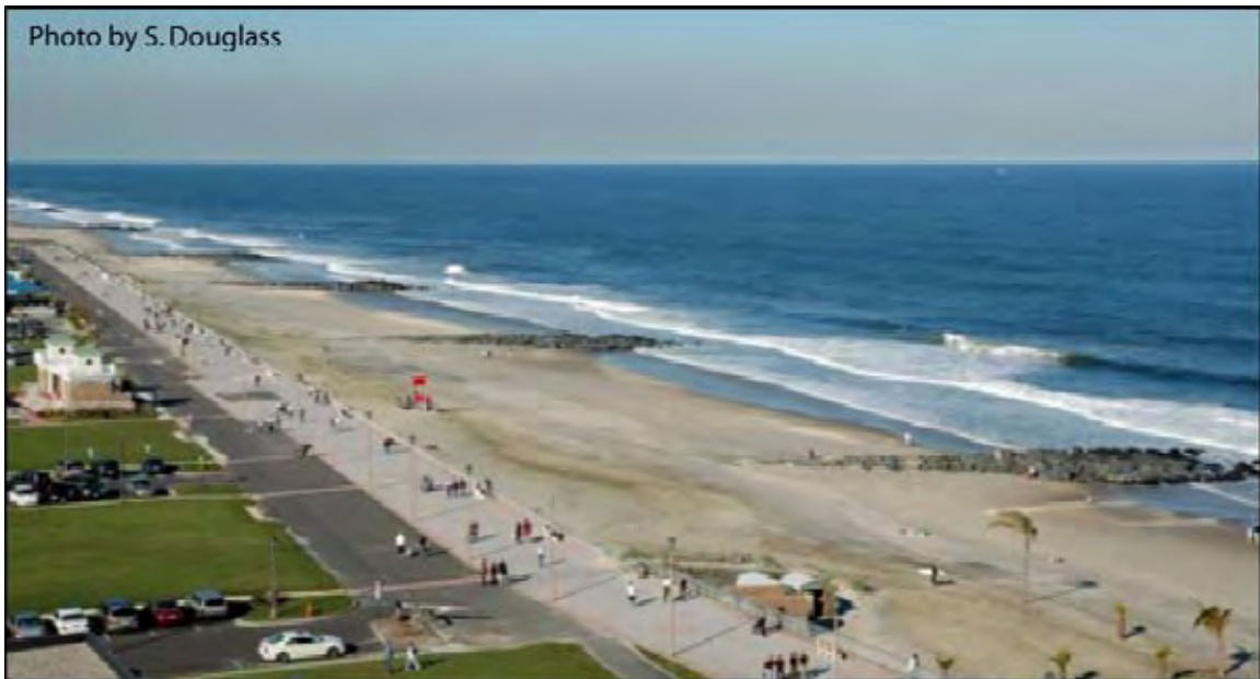
Figure 7.13. Groin field in Long Branch, New Jersey (2006)
