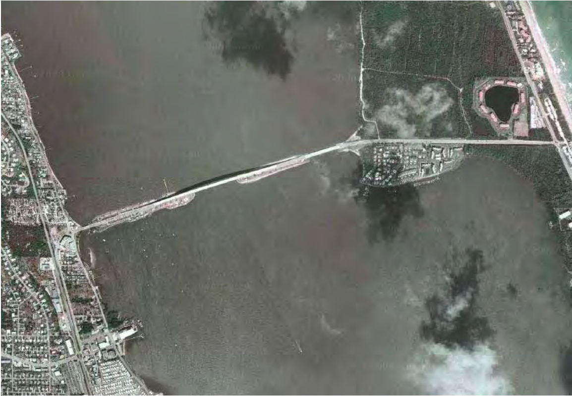
Figure 9.10. Jensen Beach Causeway bridge.
