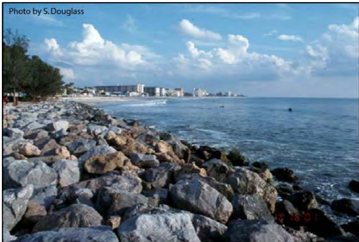
Figure 6.5. Seawall protecting a coastal highway. Venice, Florida (2001)
