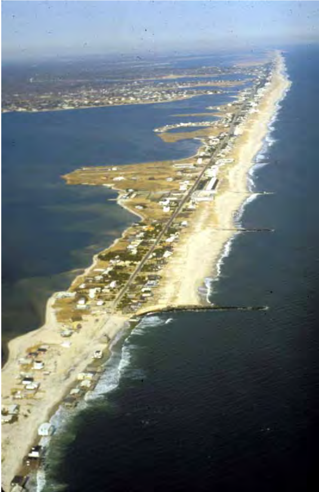
Figure 7.14. Severe shoreline recession and beach erosion downdrift of a groin field (West Hampton, New York, circa 1985, New York Sea Grant photo)
