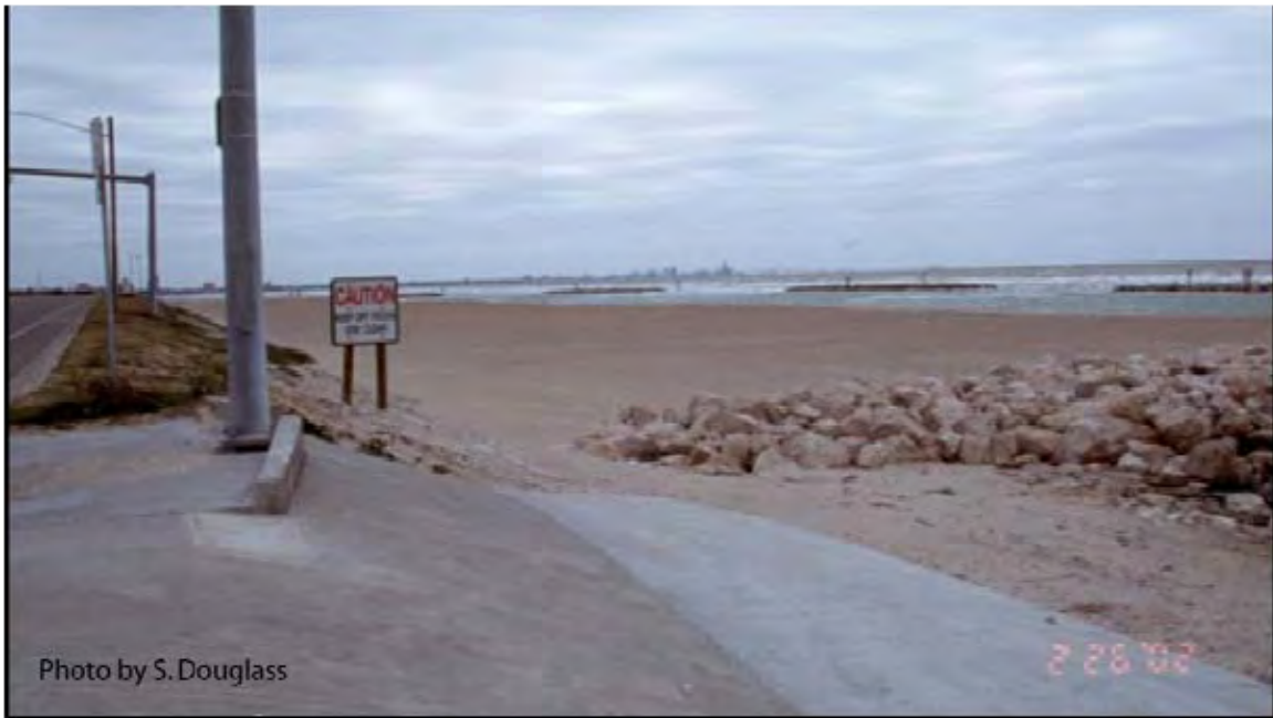
Figure 7.22. Offshore segmented breakwaters with groins and beach nourishment on Corpus Christi Bay (Ocean Drive, Corpus Christi, Texas).
