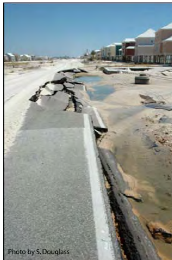
Figure 8.15. Evidence of weir-flow damage to the seaward edge of pavement due to return flow late in the storm (West Beach Blvd., Alabama 182, Hurricane Ivan, Gulf Shores, Alabama).
